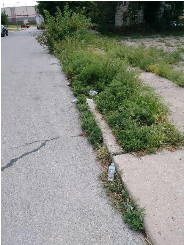
Weeds and brush in terrace, broken or missing curb
