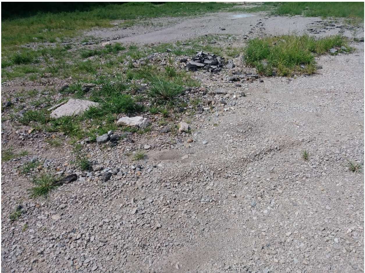
Pavement debris, weeds, uneven settling, note stormwater flow pattern
