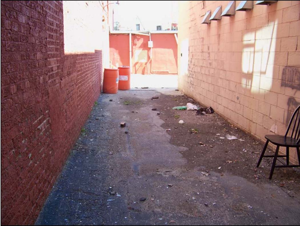
3634 Main St – looking east – poor lighting; trash/debris; graffiti
