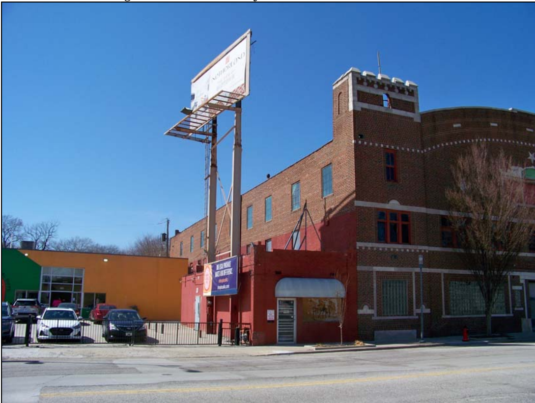
3620-3634 Main St – looking west – deterioration of windows; billboard structure
