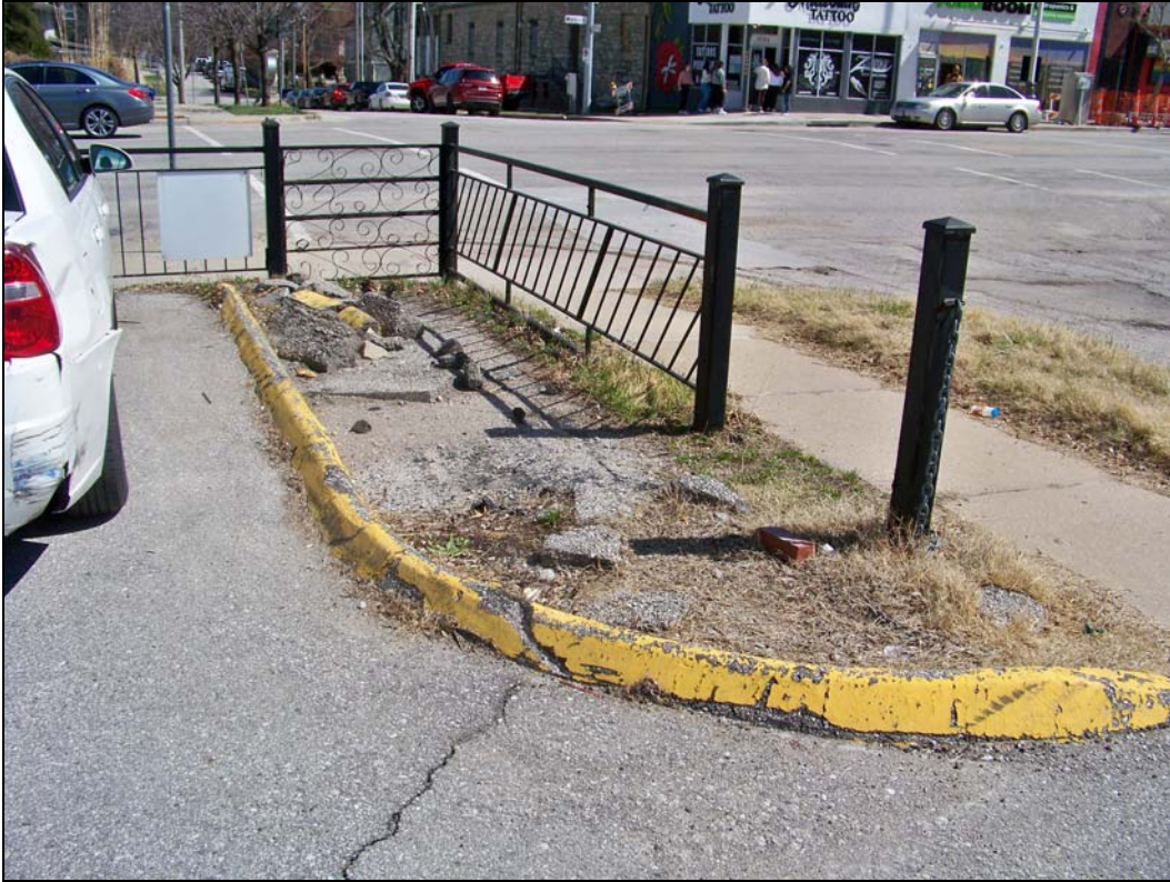
2 W. 37 th St – looking east – deterioration of fence, island; lack of landscaping
