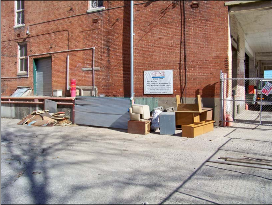
3244 Main St – looking east – trash/debris
