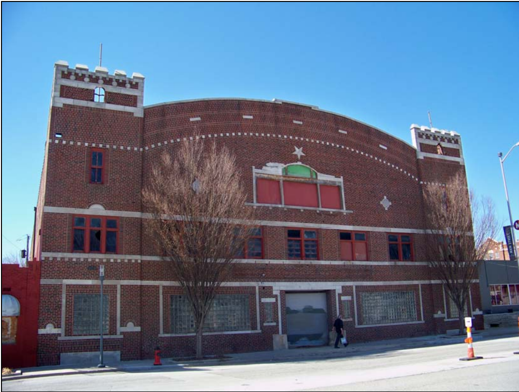
3620 Main St – looking west – deterioration of windows
