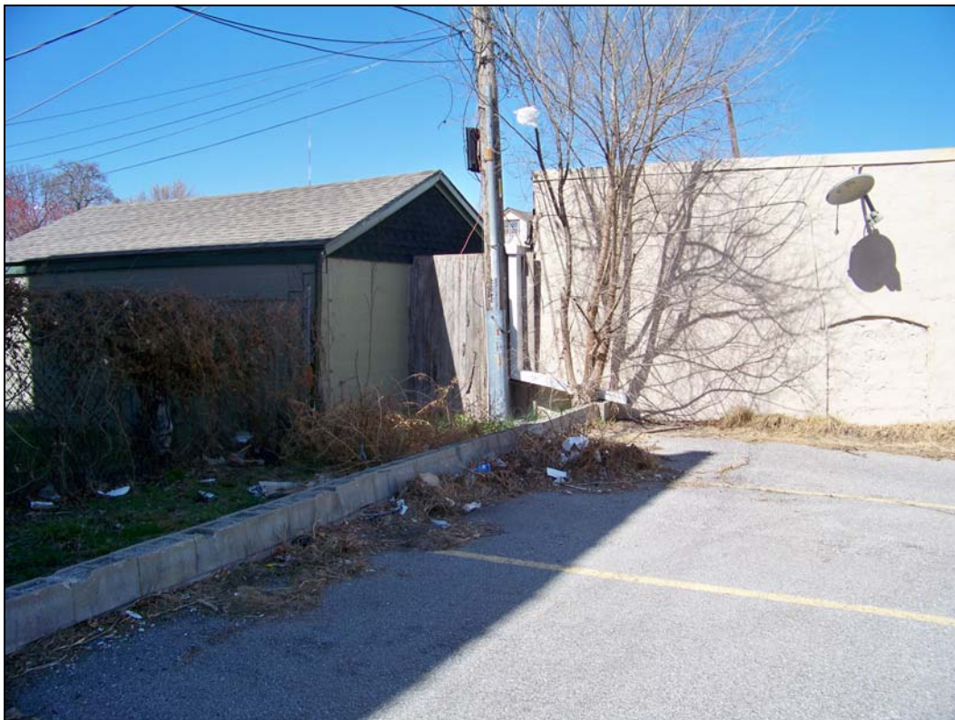
2 W 37 th St – looking north – trash/debris
