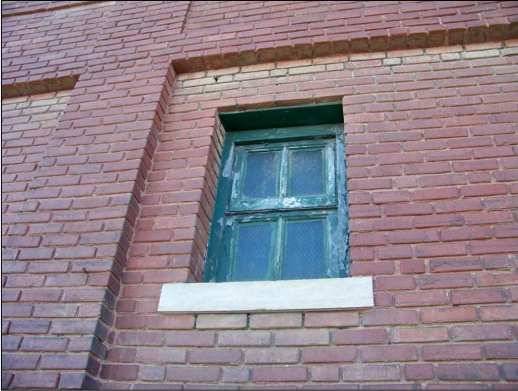
*3244 Main St – looking west – failure of finishes*
