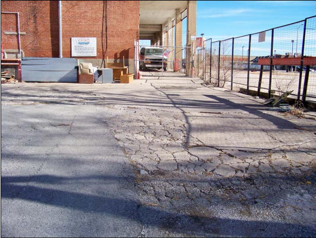
*3244 Main St – looking east – deterioration of pavement*
