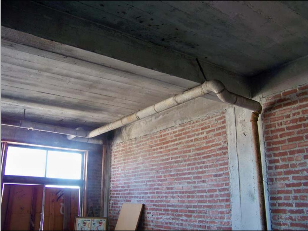
*3244 Main St – interior – asbestos pipe-wrap*
