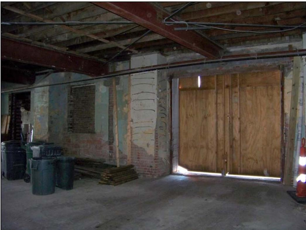
*3620 Main St – interior – deterioration of door; failure of finishes*
