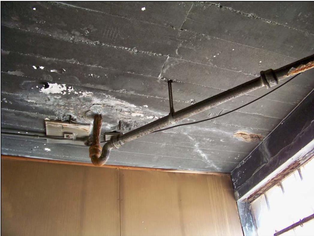
*3240 Main St – interior – deterioration of window, concrete structure, plumbing*
