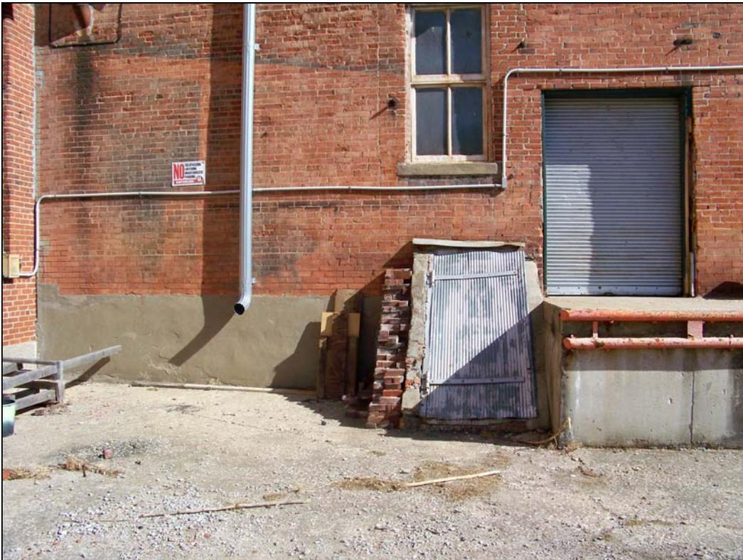
*3244 Main St – looking east – deterioration of doors, pavement; failure of finishes*
