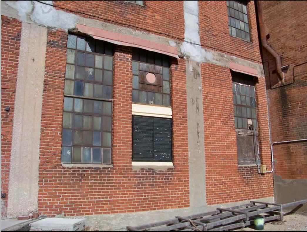
*3240 Main St – looking north – deterioration of windows, concrete structure, venting*
