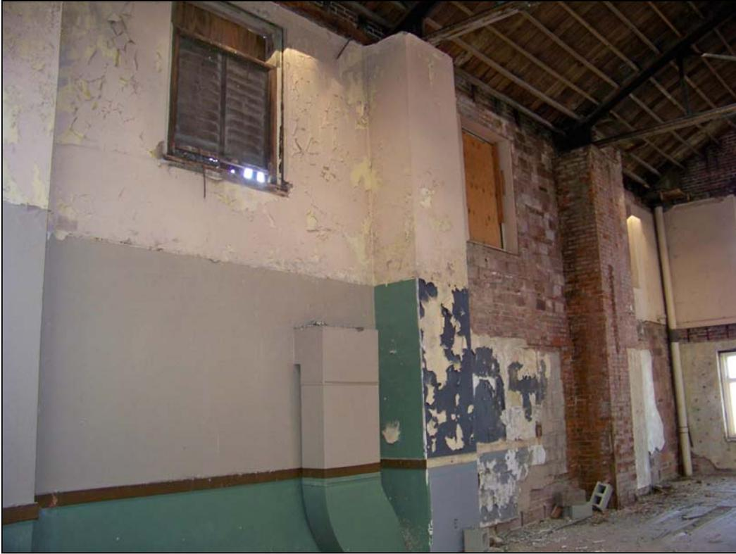
*3620 Main St – interior – failure of finishes; deterioration of windows, vents; inoperable HVAC*
