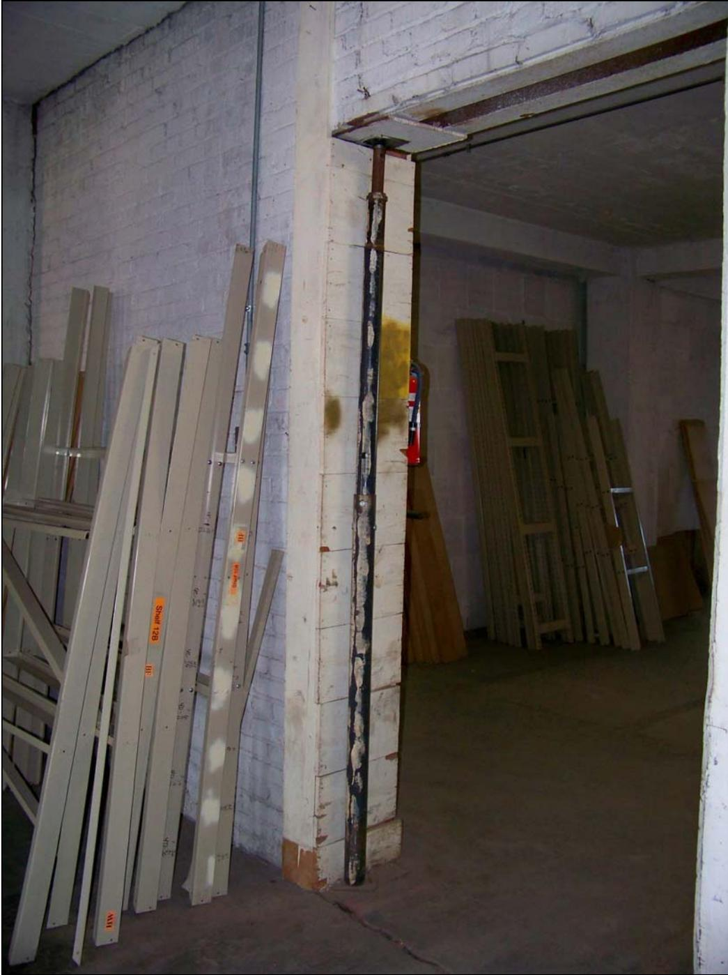
*3244 Main St – interior – deterioration of lintels; cracking of wall, floor*
