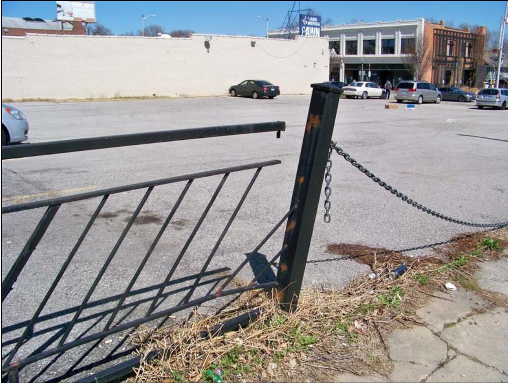
*2 W. 37<sup>th</sup> St – looking north – deterioration of fence, sidewalk*
