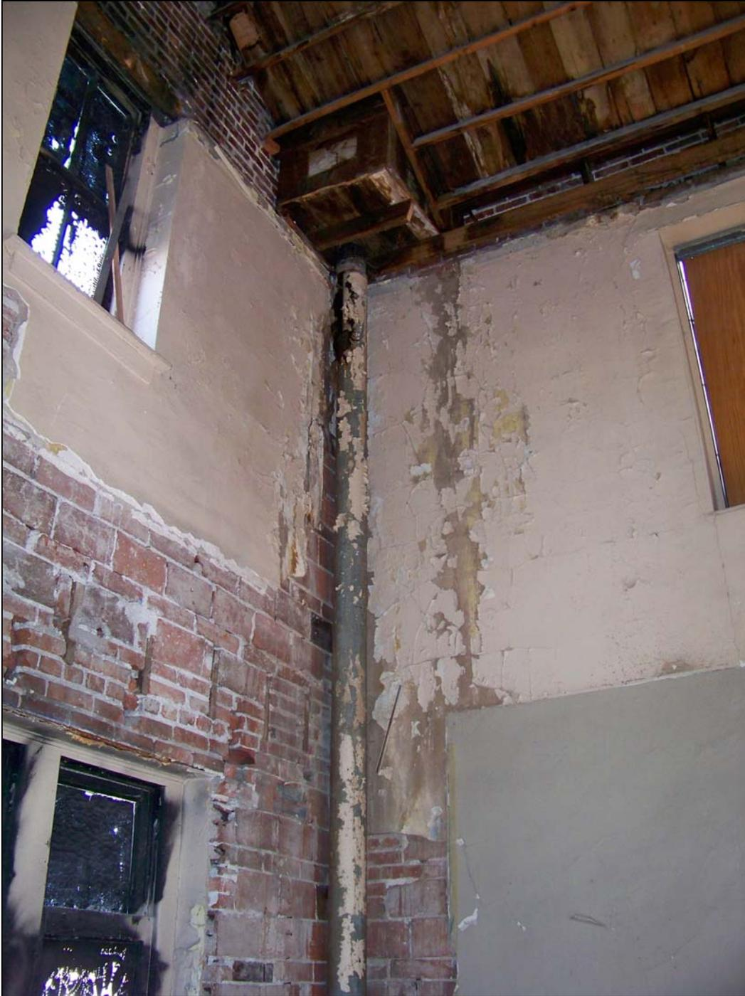
*3620 Main St – interior – deterioration of windows; failure of finishes; evidence of water intrusion*
