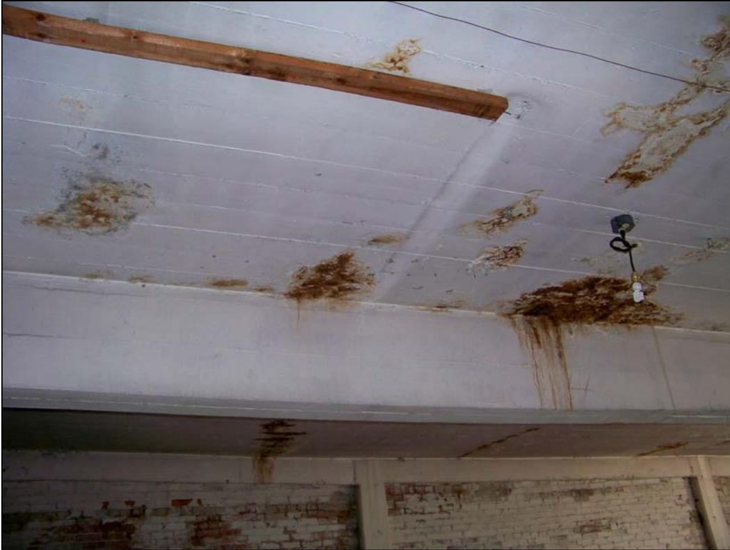
*3244 Main St – interior – deterioration of concrete structure; water damage, corroding steel rebar*
