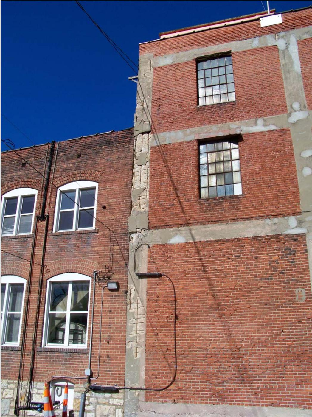
*3240 Main St – looking north – deterioration of concrete structure, windows, roof coping*
