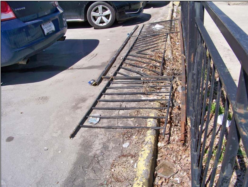
*2 W. 37<sup>th</sup> St – looking north – deterioration of fence, wheel stops*
