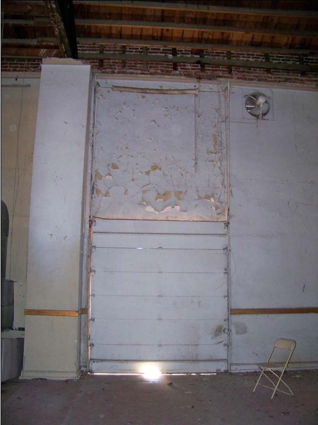
*3620 Main St – interior – deterioration of door; failure of finishes*
