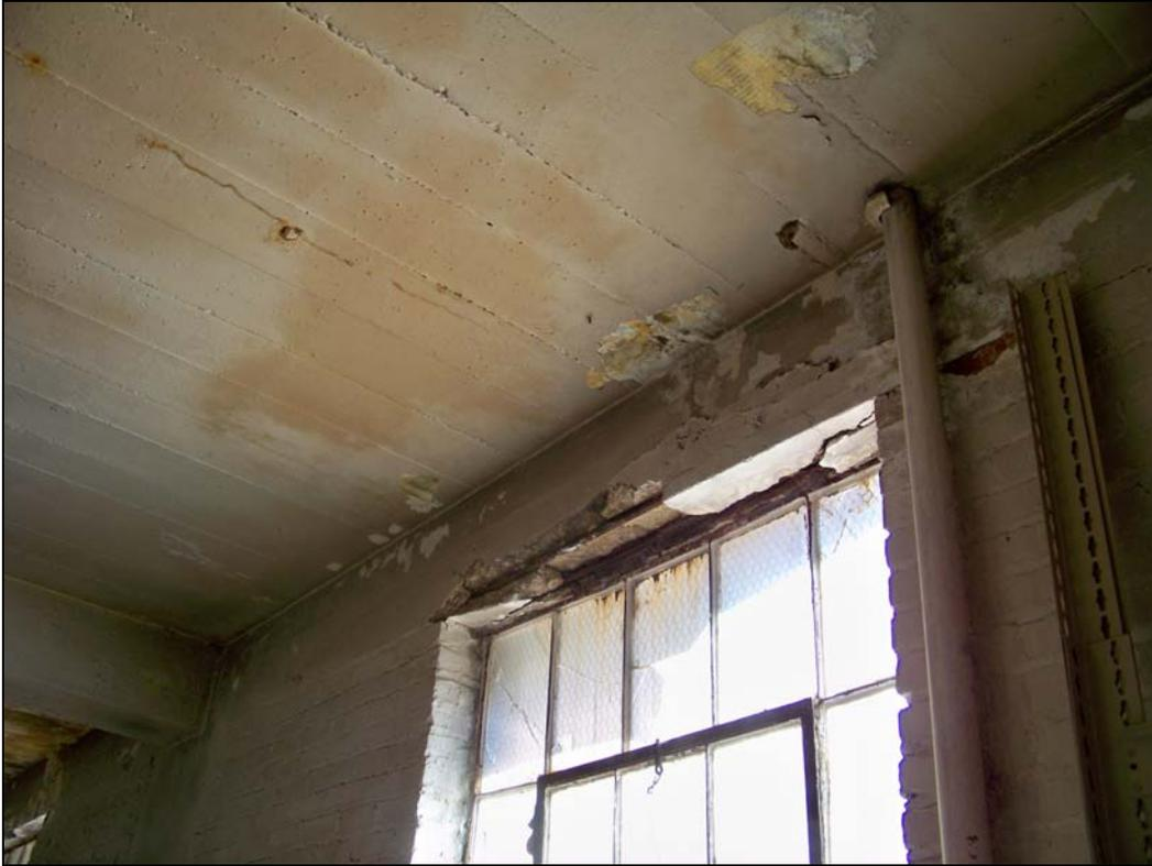
*3240 Main St – interior – deterioration of window, concrete structure*
