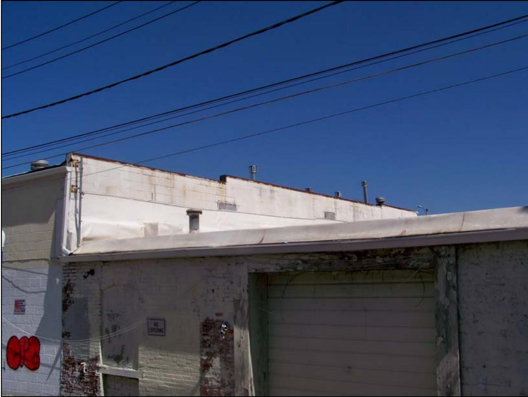
*3634-3636 Main St – looking north – deterioration of roof coping; failure of finishes*
