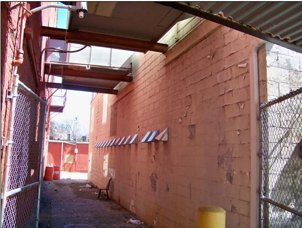
*3634 Main St – looking east – failure of finishes*
