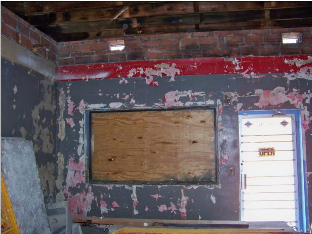
*3620 Main St – interior – deterioration of windows; failure of finishes*
