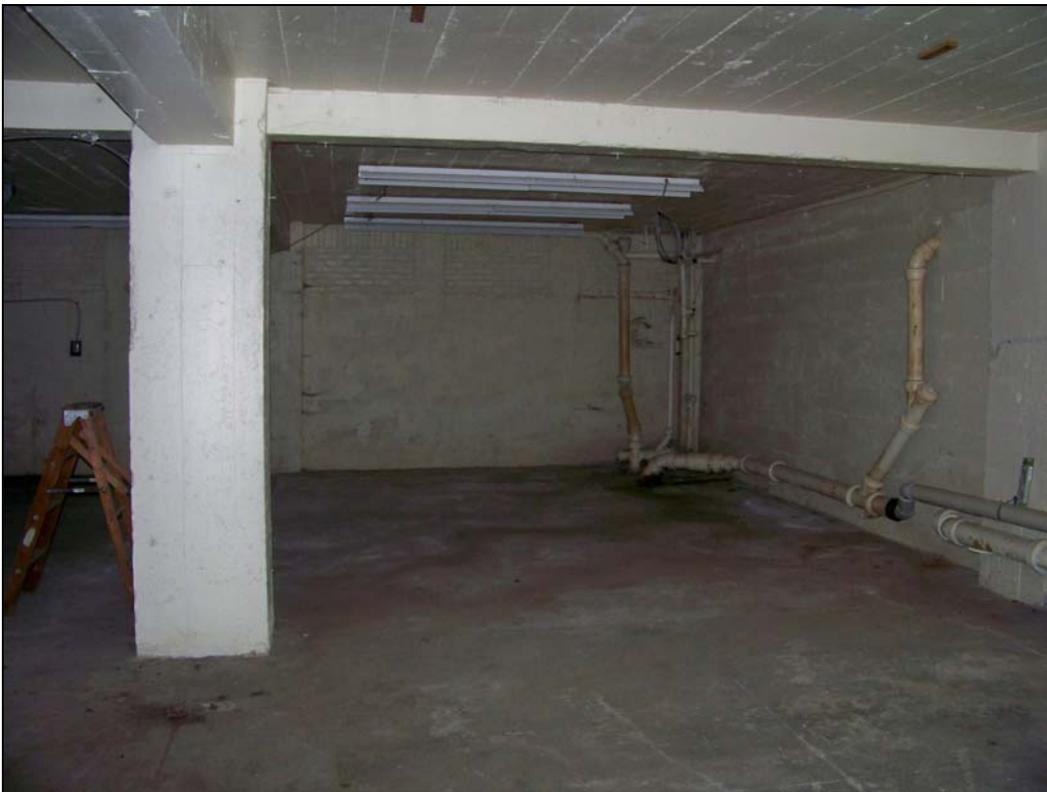
*3240 Main St – interior – leaking plumbing and staining of floor*
