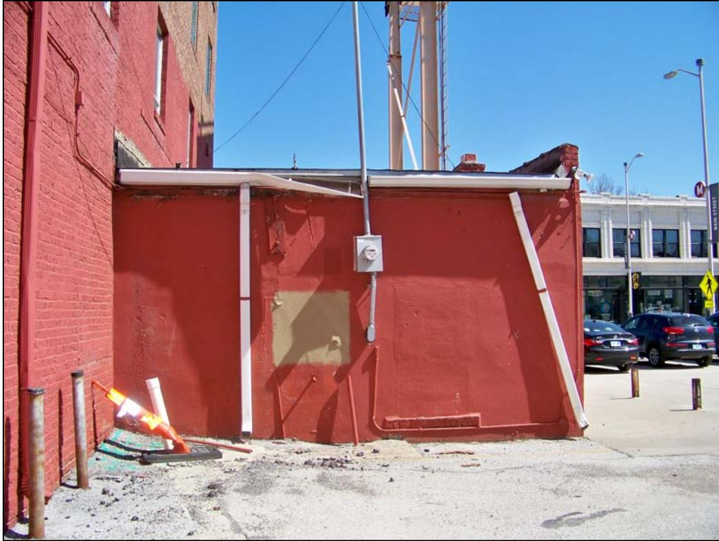
*3634 Main St – looking east – deterioration of gutter, downspouts; failure of finishes*
