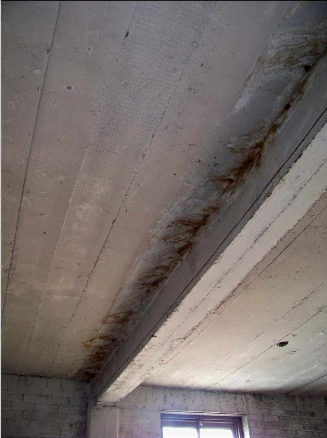
*3244 Main St – interior – deterioration of concrete structure; water damage, corroding steel rebar*
