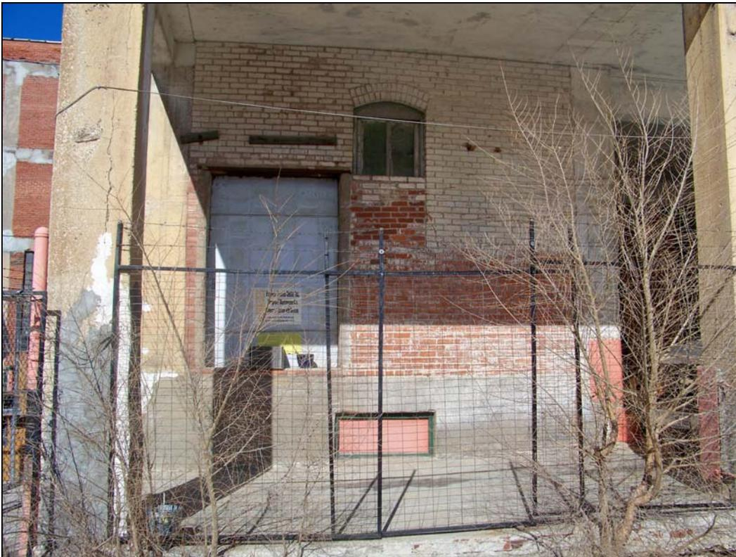
*3244 Main St – looking north – failure of finishes; deterioration of door, windows*
