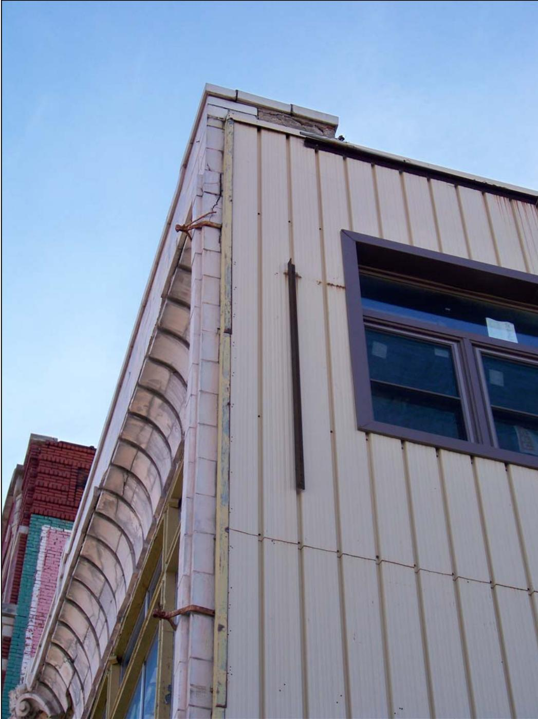
*3240 Main St – looking southwest – deterioration of terra cotta; failure of finishes*
