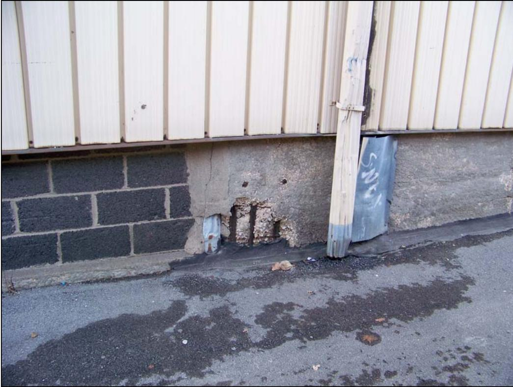
*3240 Main St – looking south – deterioration of wall, downspout*
