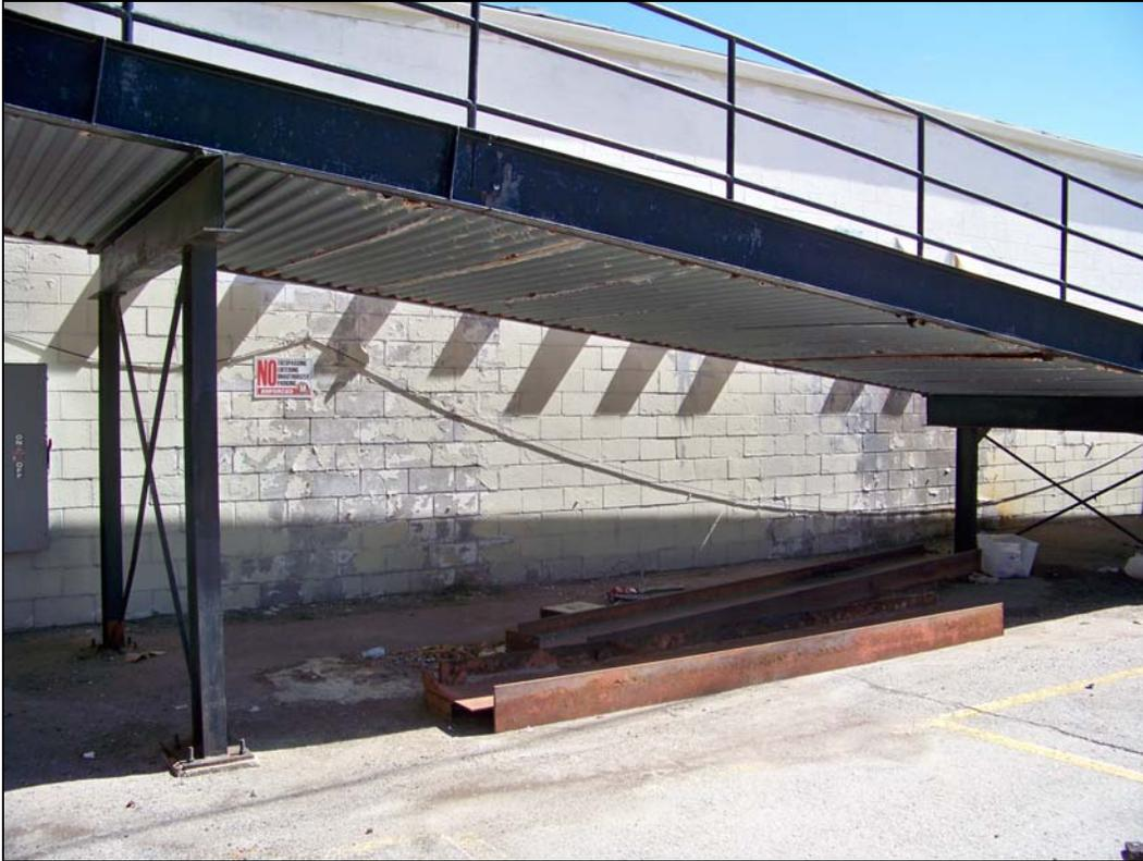
*3634 Main St – looking east – failure of finishes; corrosion of ramp structure*
