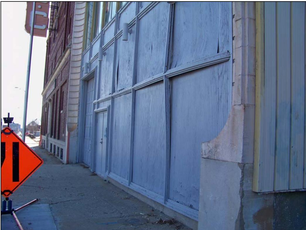
*3240 Main St – looking south – deterioration of wall; failure of finishes*
