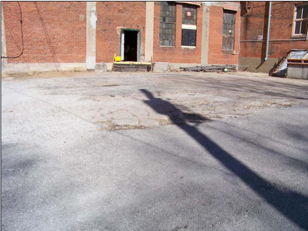
*3244 Main St – looking northeast – deterioration of pavement*
