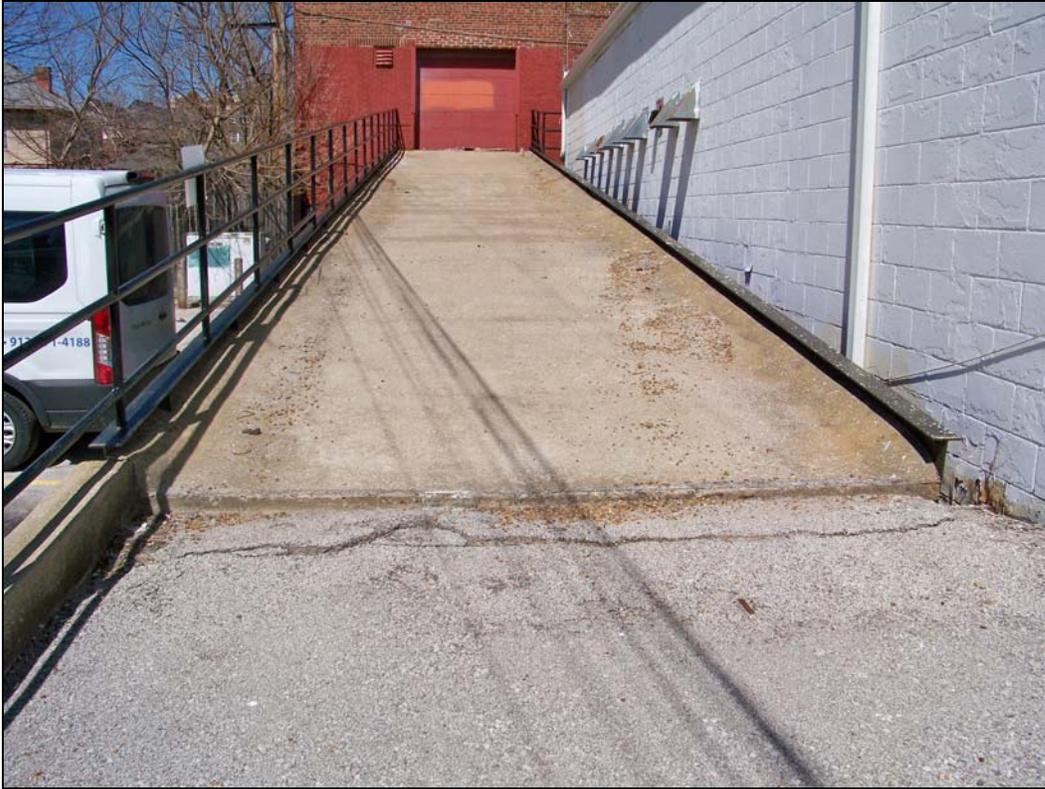
*3634 Main St – looking north – deterioration of pavement*
