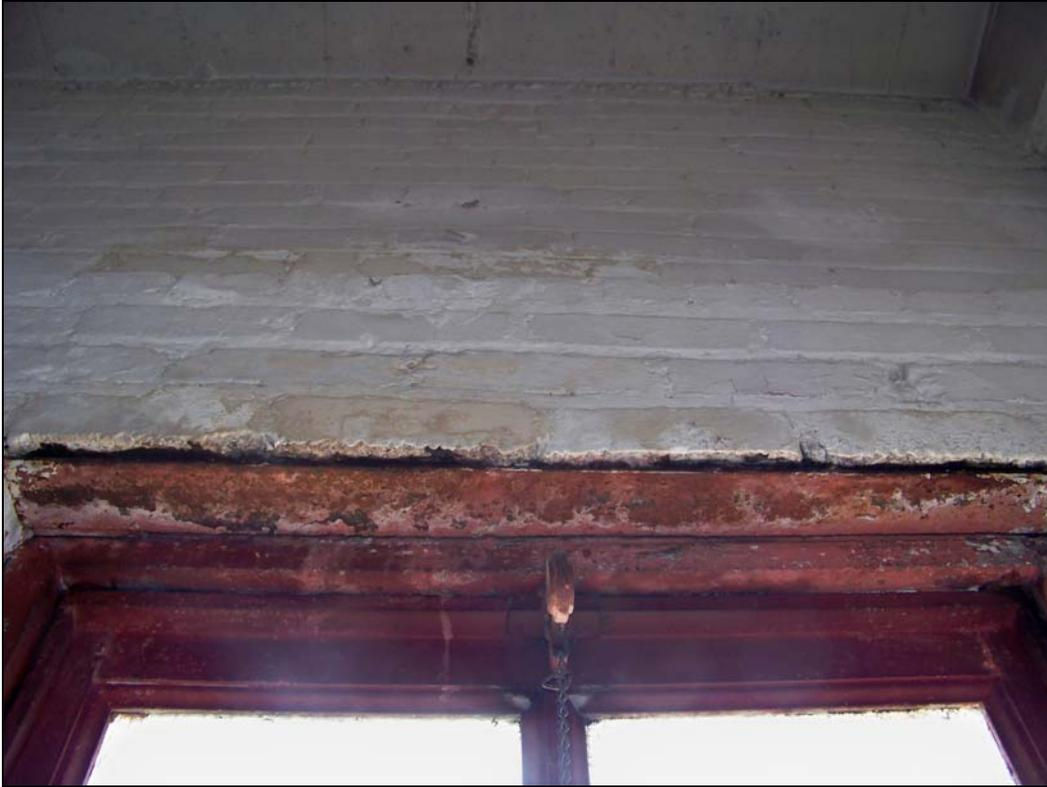
*3244 Main St – interior – deterioration of window, lintel; failure of finishes*
