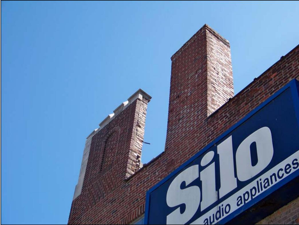
*3620 Main St – looking south – deterioration of parapet wall, mortar, masonry*
