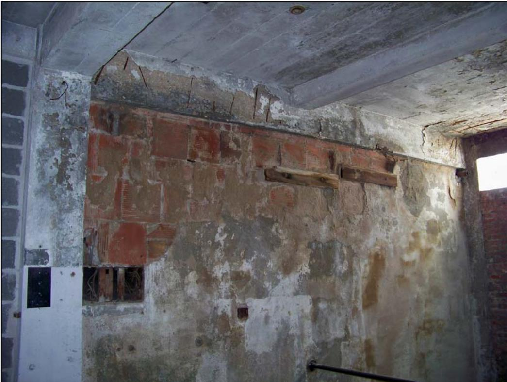
*3240 Main St – interior – deterioration of concrete structure, wall; failure of finishes*
