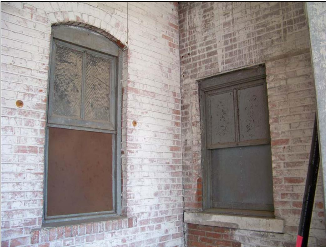
*3244 Main St – looking northeast – deterioration of windows; failure of finishes*
