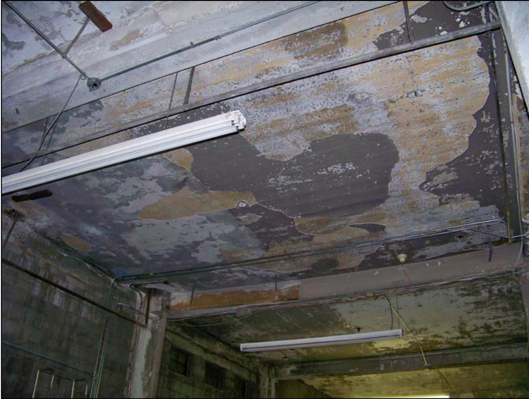
*3240 Main St – interior – failure of finishes*
