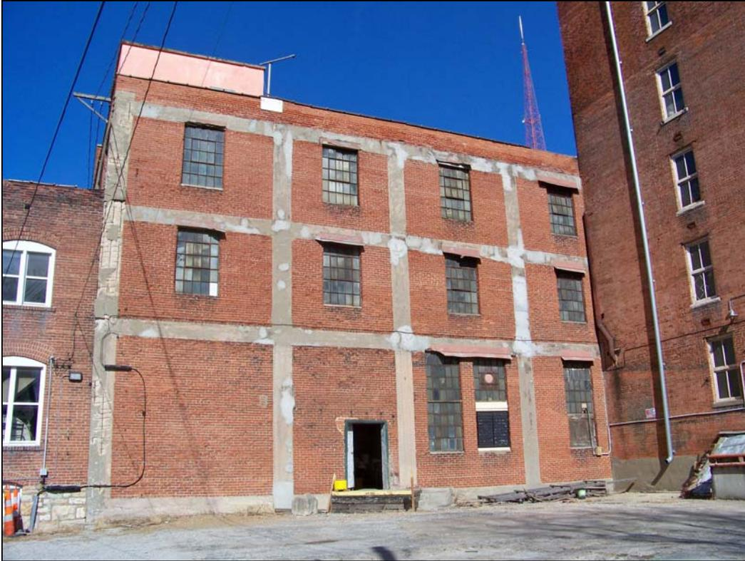
*3240 Main St – looking north – deterioration of windows, concrete structure*
