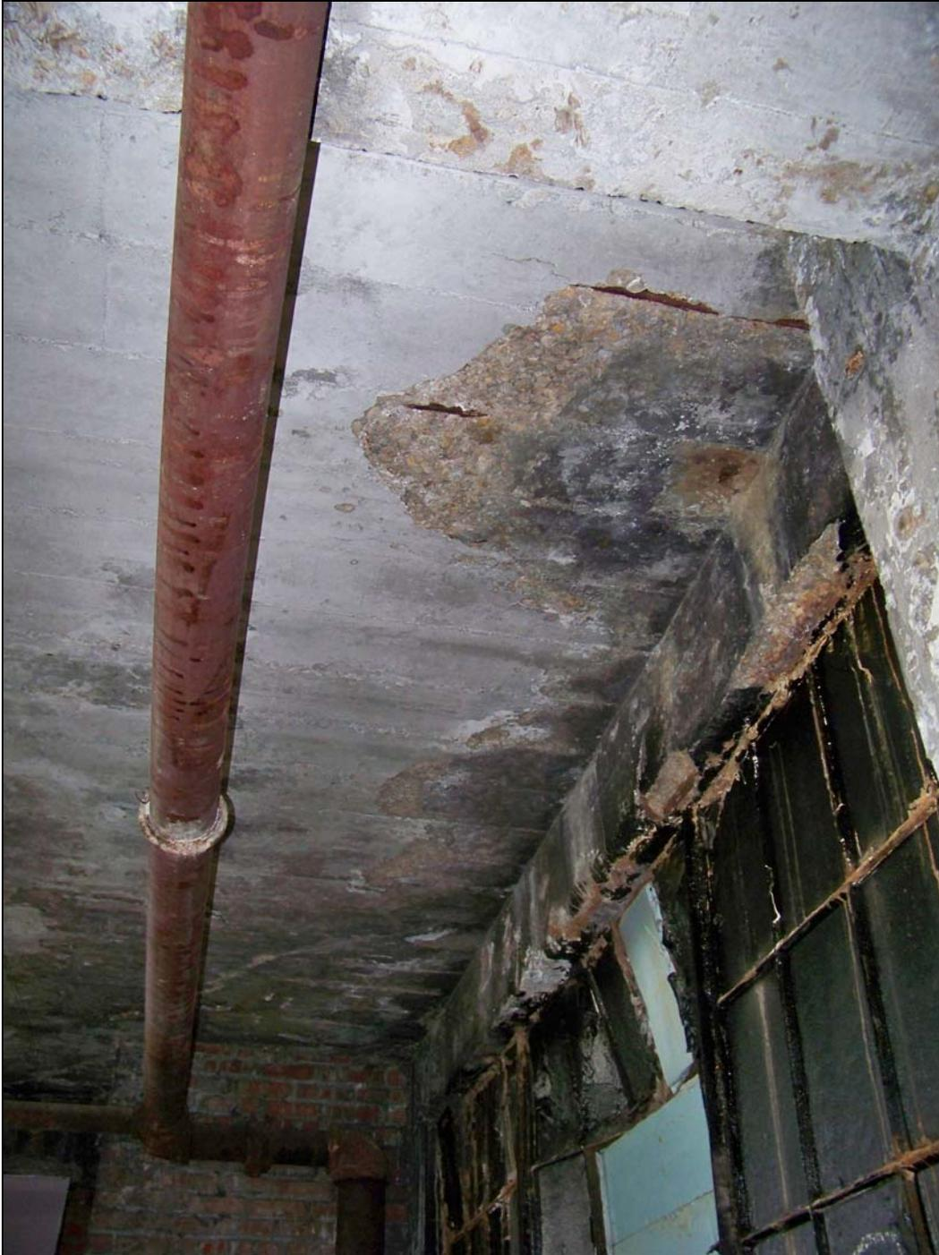
*3240 Main St – interior – deterioration of window, concrete structure, plumbing*
