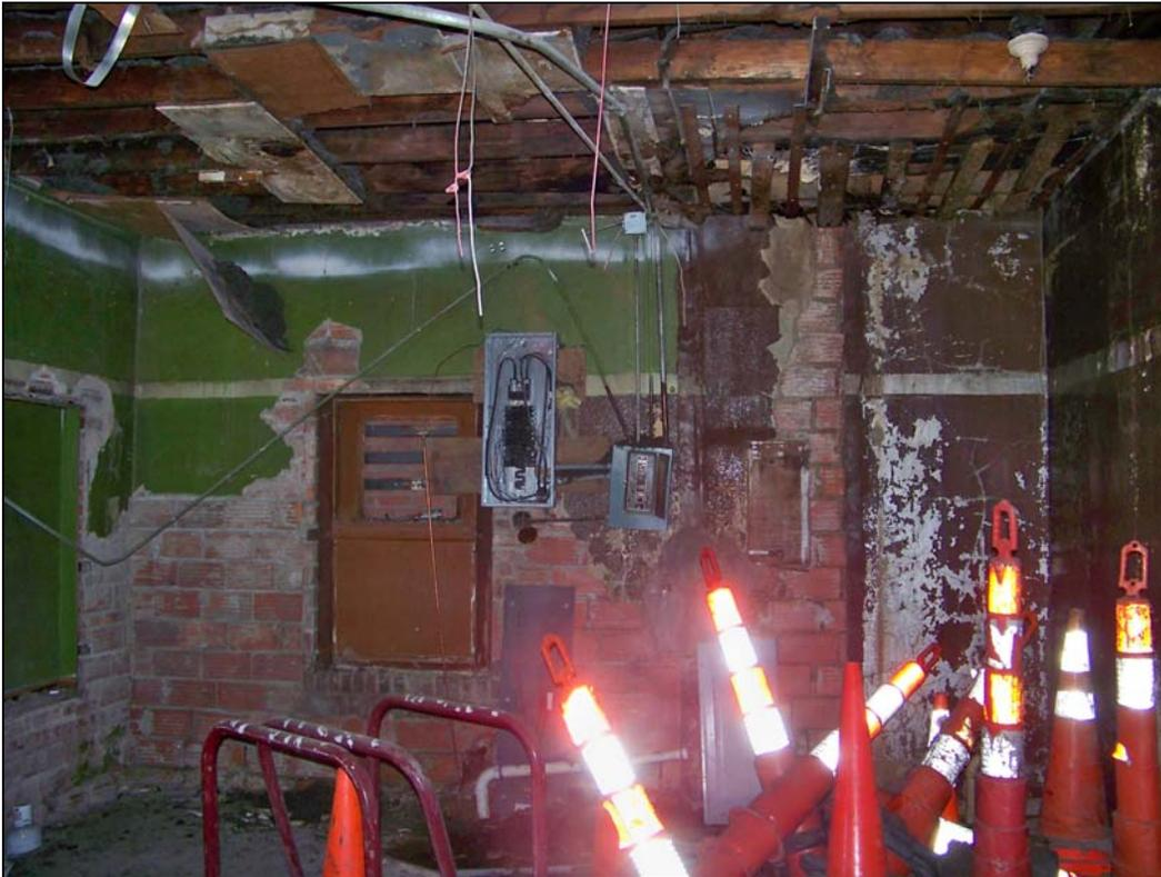
*3634 Main St – interior – inoperable building system; deterioration of ceiling, wall coverings, finishes*
