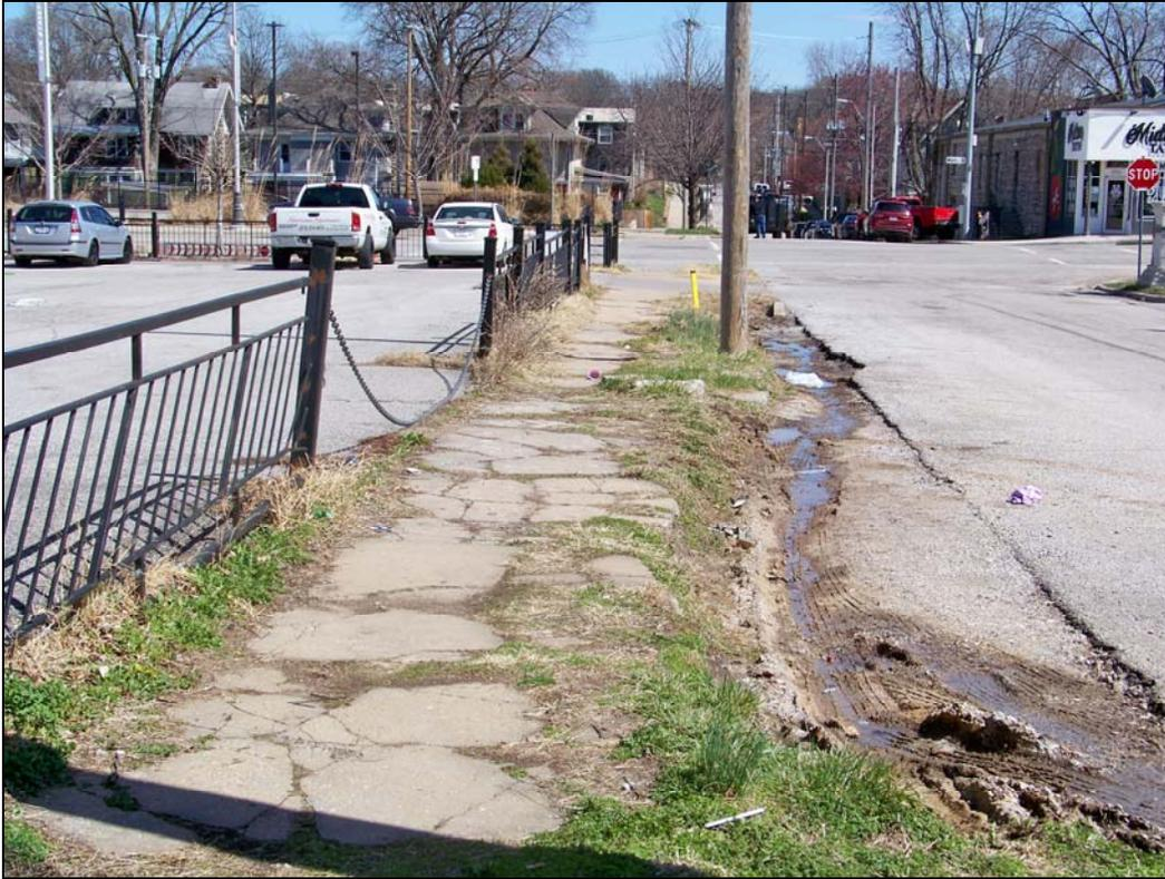
*2 W 37<sup>th</sup> St – looking east – cracked/uneven sidewalk and curb*
