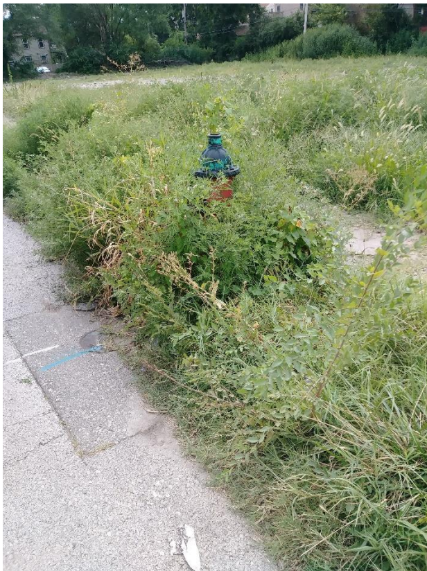
Weeds; note poor visibility of fire hydrant
