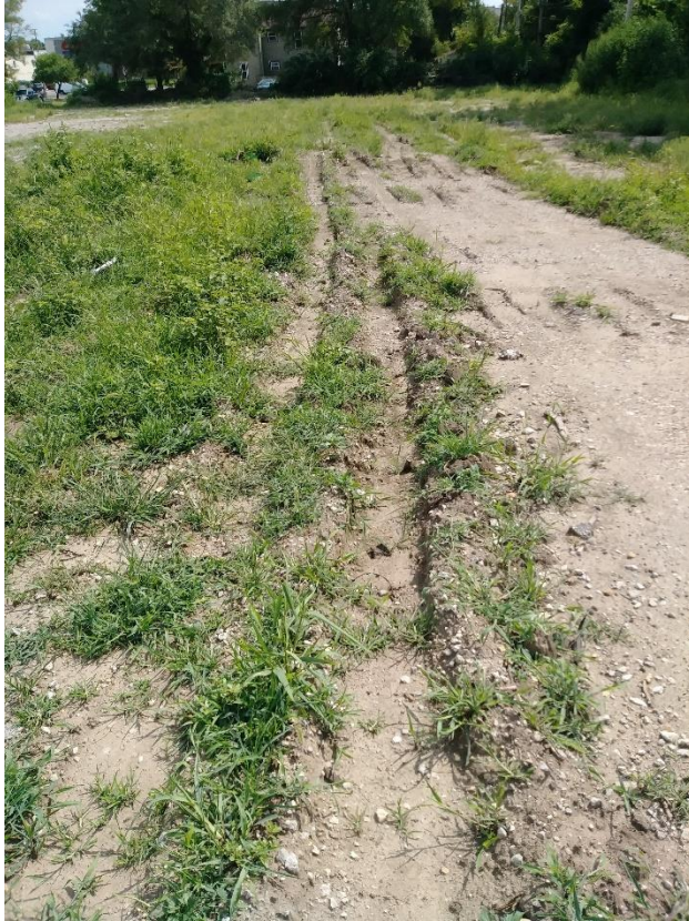
Ruts from vehicles in unpaved surface
