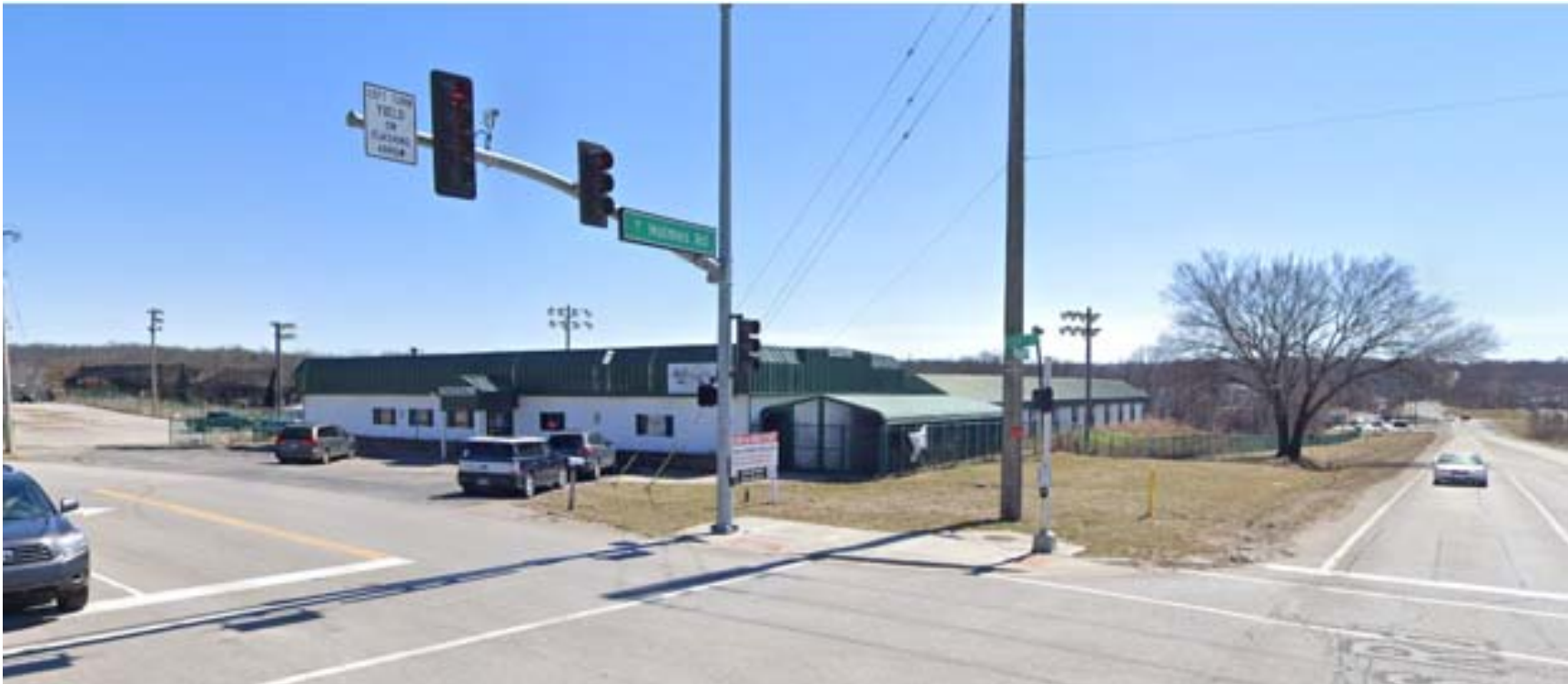
Looking southeast from intersection of 135 th Street & Holmes Road
