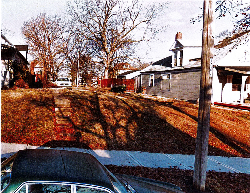
2538 Olive Street – note deteriorating stairs, illegally parked truck
