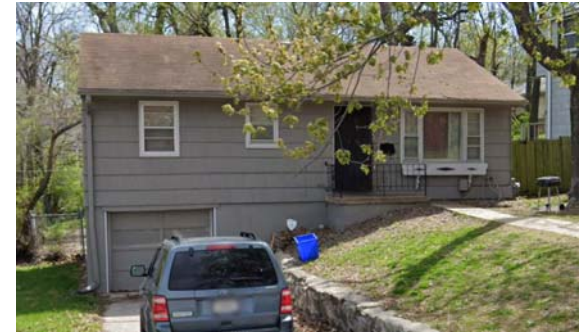
1907 E. 79 th Street Roof repair
