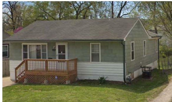
8330 Park Avenue Roof repair
