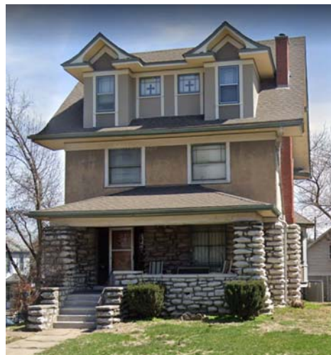
2601 Charlotte Painting, window and gutter replacement
