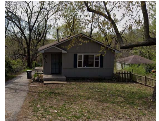
8240 Wayne Avenue Roof repair
