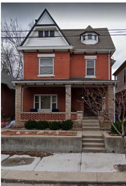
500 Olive HVAC and roof repair
