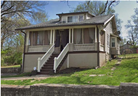
2005 E. 81 st Street Roof repair
