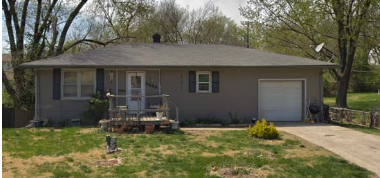
8444 Wayne Avenue Roof repair
