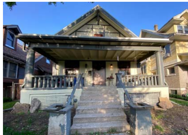
3023 Campbell Painting, siding and gutter replacement
