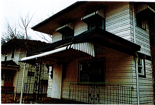
4105 College Ave. Exterior and interior repair
