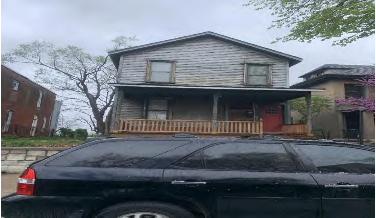
Figure 11. 1616 Madison Ave. House in disrepair.
