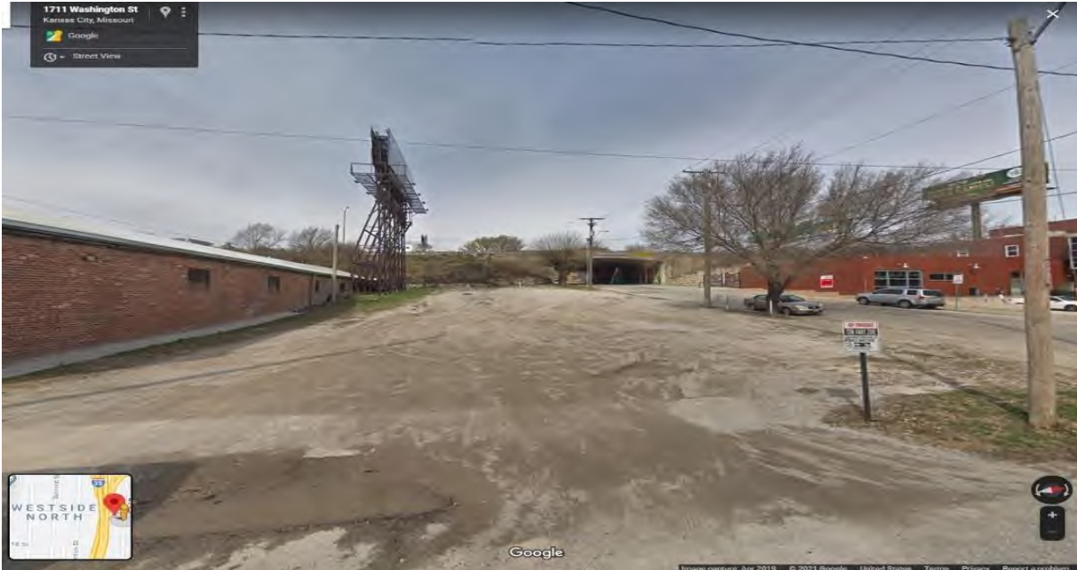
Figure 1. 503 W. 17 th St. Unimproved lot with poor drainage.
