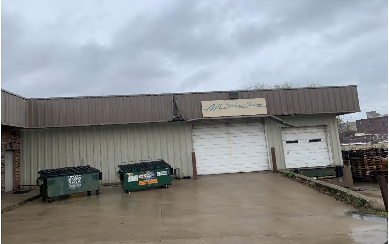
Figure 18. 2001 W. Pennsylvania Ave. Damaged building and unsecured wood pallets.
