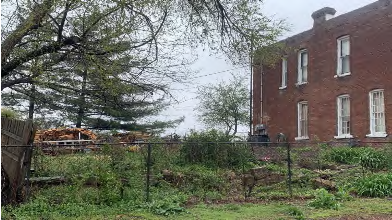
Figure 7. 802 W. 16th St. Large woodpiles in overgrown yard present a fire hazard.
