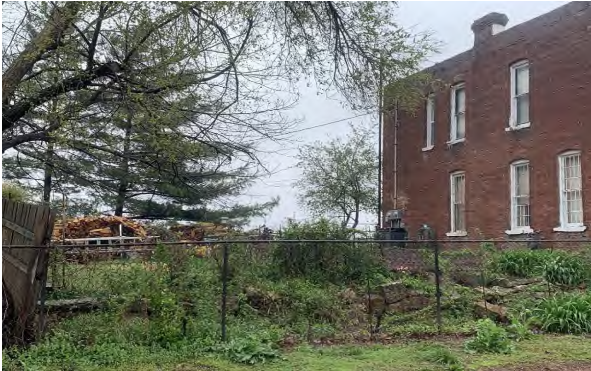
Figure 6. 802 W. 16th St. overgrown brush and oversized woodpile.
