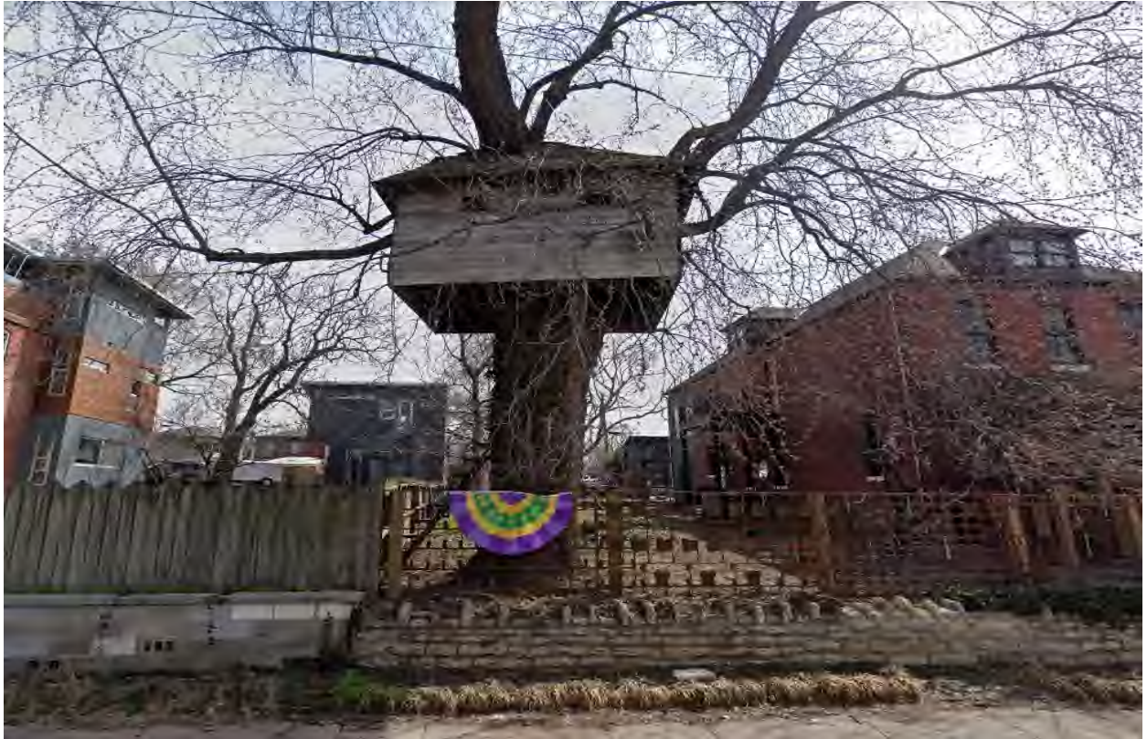
Figure 6. 1644 Madison Ave. Dilapidated tree house hanging over sidewalk.
