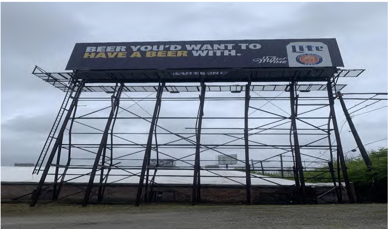
Figure 2. 17th St. and Washington. Southwest corner billboard.
